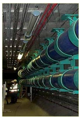
Pipes diverted into an old tunnel ( $\ensuremath{\mathbb{C}}$  Metronet Rail SSL Ltd / created by Allies and Morrison)
