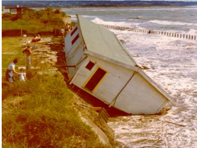
Figure 1.1: Effects of coastal erosion adjacent to a tidal inlet. (Note railway-iron stakes offshore – an earlier attempt to protect shoreline.) [Source: R.K. Smith].
