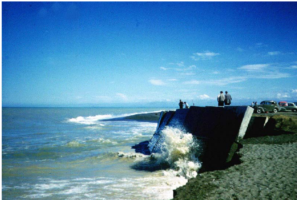
Figure A3.2: Attempted armouring of the gravel/sand beach at the mouth of the Orari River, South Canterbury (late 1950s). ( Source: D. Todd).
