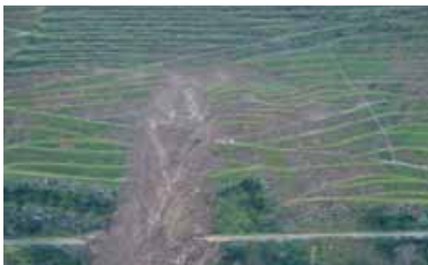
Road removed by a landslide. Villa Real district, Portugal Source: Nuno Cristelo
