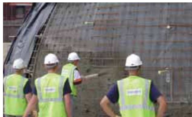
Shotcrete application Source: Shotcrete Services Ltd
