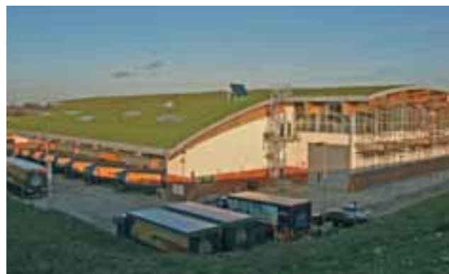
Adnams Brewery Warehouse, Suffolk Source: Lime Technology
