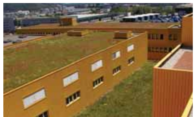
The Schachermayer factory green roof in Linz, Austria Source: Municipal Planning Board of Linz
