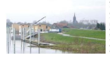
from floating off during a flood, they are anchored to flexible mooring posts that cushion the swell of the water. It is expected that, once every five Houses that float during floods...
