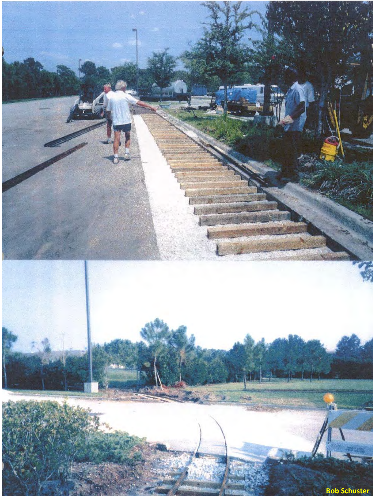
Figure 5 Very inexpensive narrow gauge rail track installation
