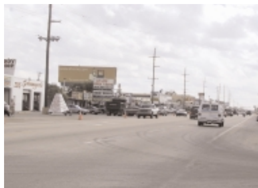
The State Road 7 Collaborative is working to transform areas such as this.
